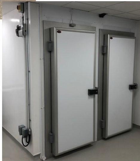
-30°C freezer system and 3°C Fridge installation
